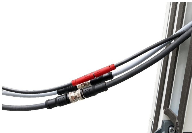
Fig. 39: Connection of the cables
